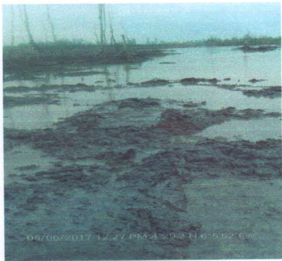
Fig D: picture taken after backfilled
