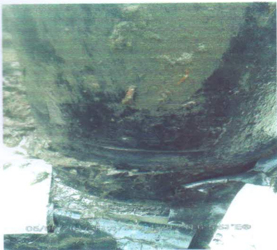
Fig B: picture taken after excavation
